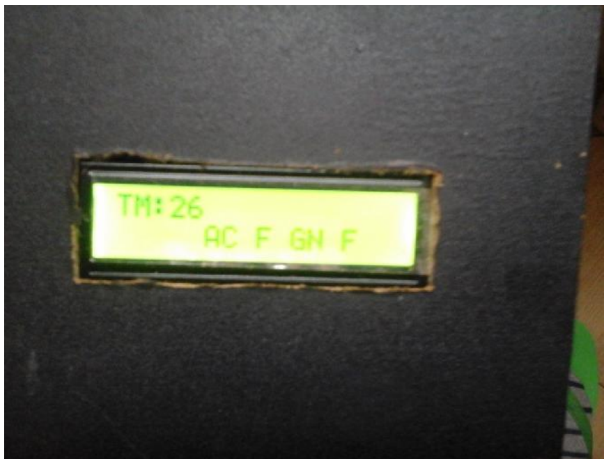
Fig. 5.13. Screenshot showing temperature, AC and Generator failure.
